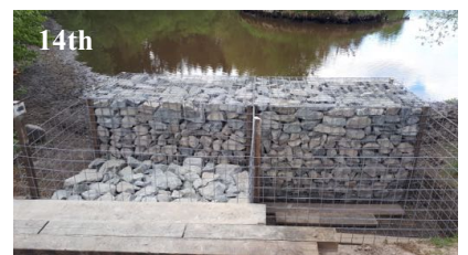
Treated ramp of Red Squirrel Hide and started filling basket 3.
