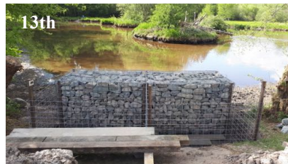
Erected baskets 3 & 4 and prepared for filling.
