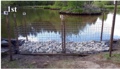
Added third layer of stones to gabion baskets 1 and 2.
