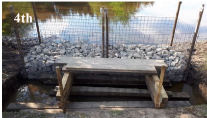
Added stones and strengthening cables.
