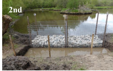
Dug out the area for gabion baskets 3 and 4.
