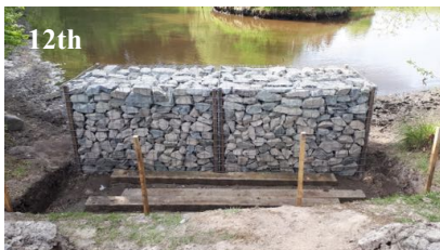
Completed filling baskets 1 & 2 and tied down the lids.
