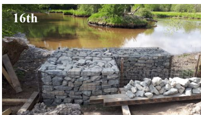
Completed basket 3 and started on 4.
