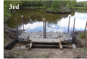
Constructed platform for transferring gabion stones.
