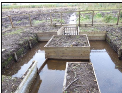
Silt trap rebuilt
