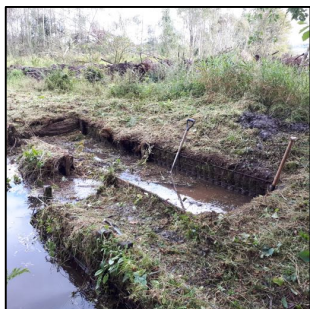
Silt trap damaged
