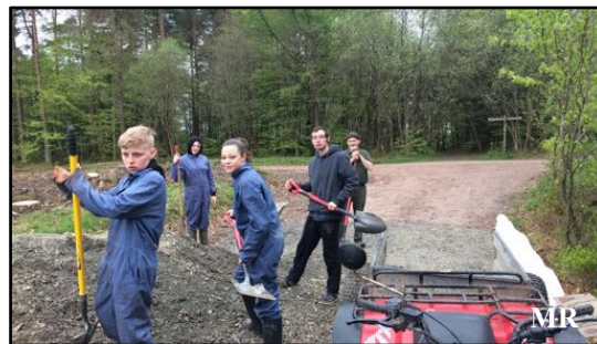
Laying gravel path using quad bike and trailer
