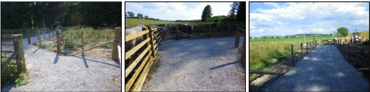
Day 9. Part of fence between area of Hunting gate and Wood gate fenced off. Field gate erected and area made stock-proof.
