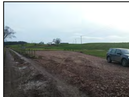
6th. Stone foundation complete.
