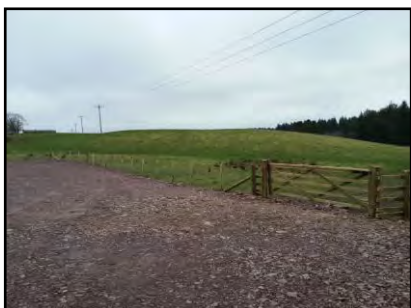
19th. Field gate erected.
