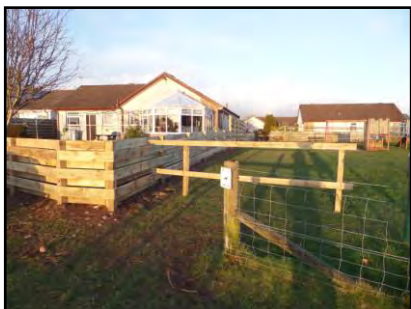
7th. Safety barrier erected at Isle Court children's play park.
