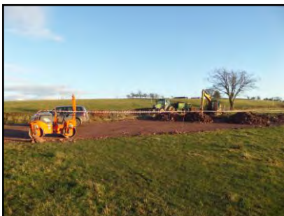
4th. Stone base laid and rolled.
