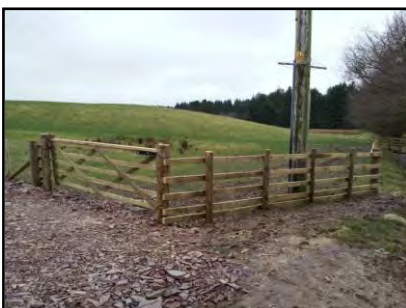
19th. Wooden fence erected at field gate.
