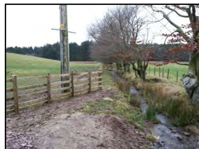
19th. Wooden fence erected at field connection.
