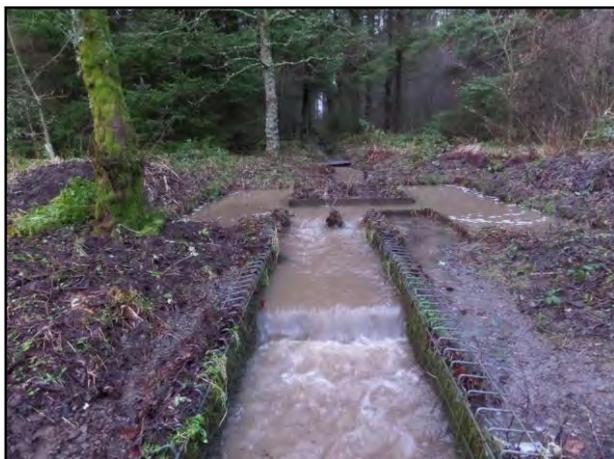
2<sup>nd</sup> - High water level in the silt trap
