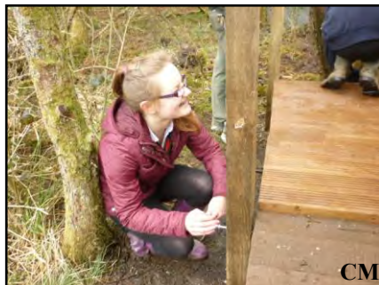
Pamela Beeton inserting the coach bolts.
