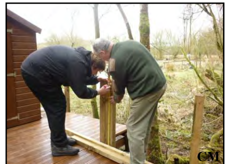
Danny Brannan measuring and marking posts.
