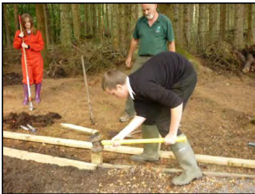
5. Hammering in posts
