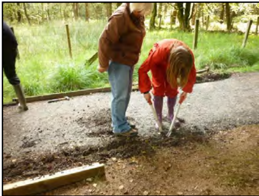
3. Cutting tree roots as necessary
