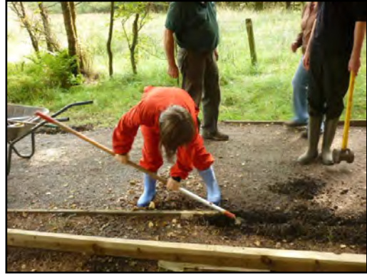
2. Digging channel for new board
