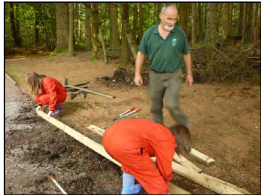
4. Putting new board in place
