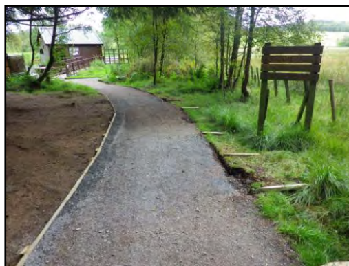
7. Posts trimmed and path edge filled with gravel to finish the section
