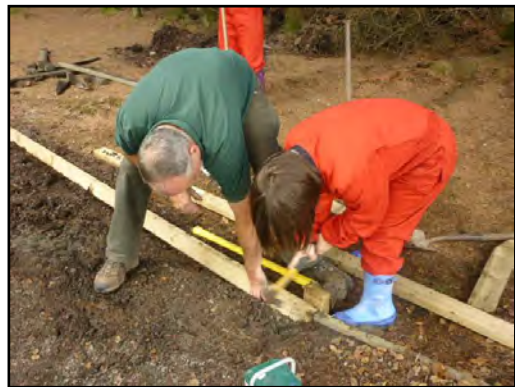
6. Nailing board to posts
