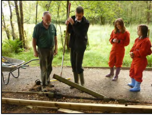
1. Removal of old board
