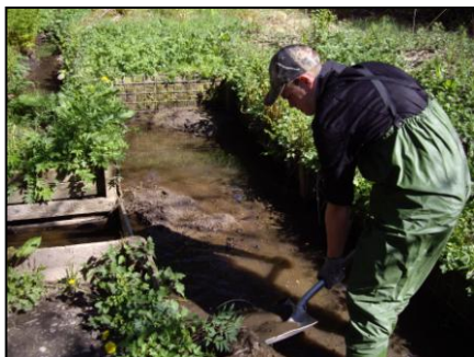
Chris Trott clearing silt trap 01.05.11
