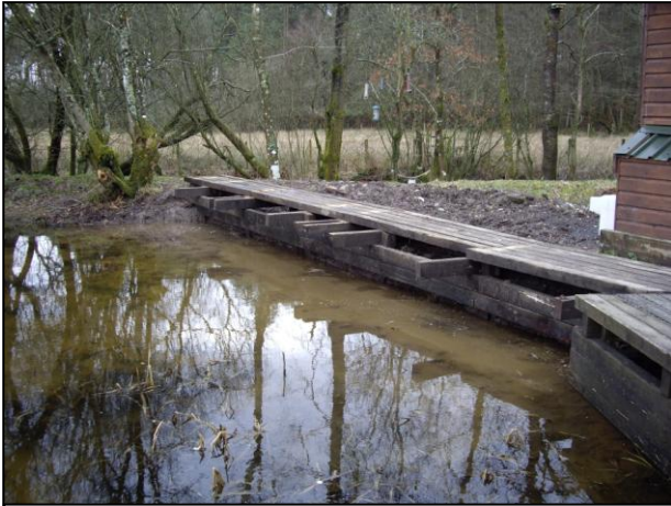
The facing was completed on 18th February.
