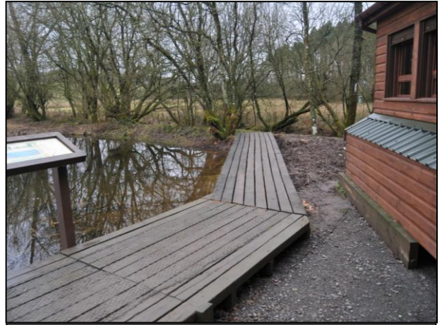
The top was completed on 19th February.
