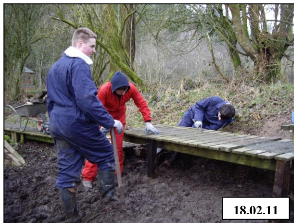
Pupils helping to raise mid-section of boardwalk.
